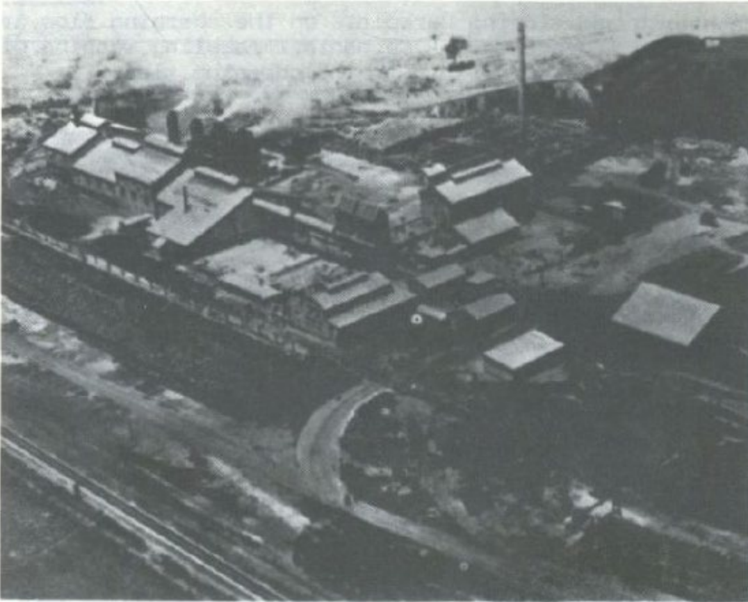
Figure 6 : Newnam Hearth Plant 1946 with sinter beds top right, and cupola type furnace stacks top left.
